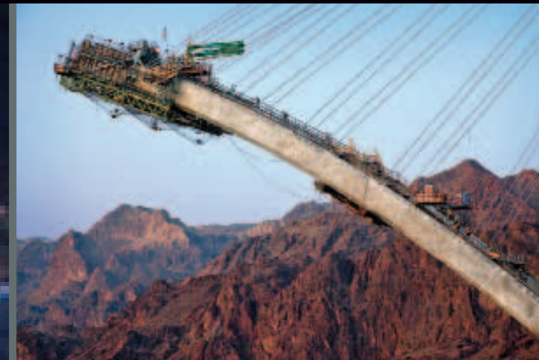
Just as they did every morning, ironworkers climbed up the Nevada side of the arch segment on April 29, 2009, to start work. Cable stays supported the arch construction until the arch span was completed.
