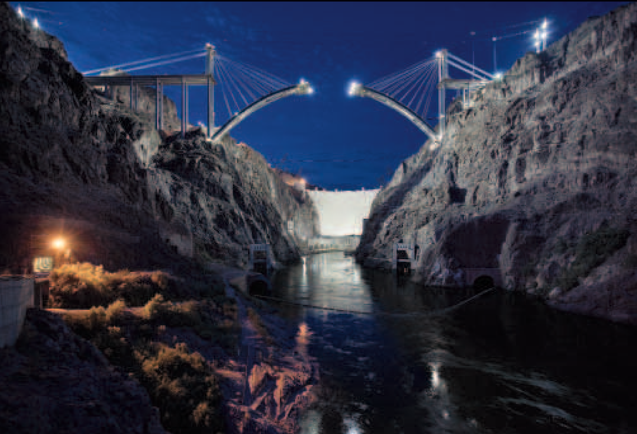
Captured from the banks of the Colorado River on May 21, 2009, this image features the 24-hour construction of the arch as concrete was poured at night to take advantage of cooler temperatures.
