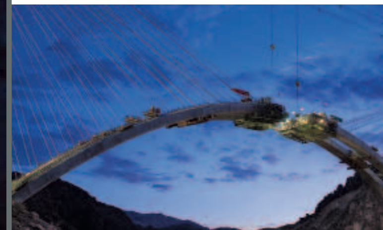
On the evening of June 29, 2009, the Arizona and Nevada arch segments neared their rendezvous point over the Colorado River.
